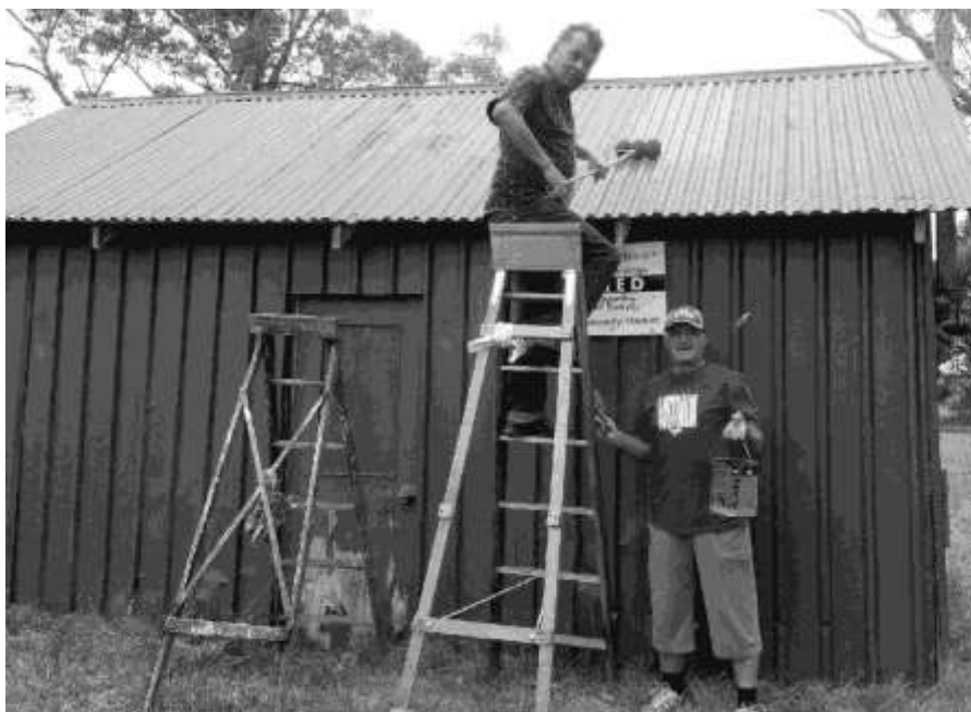
Photo: (L-R) Arthur Porter rolling paint on to the roof of the shed as Tony Arrigo steadies the ladder and assists painting the external wall with a brush.
